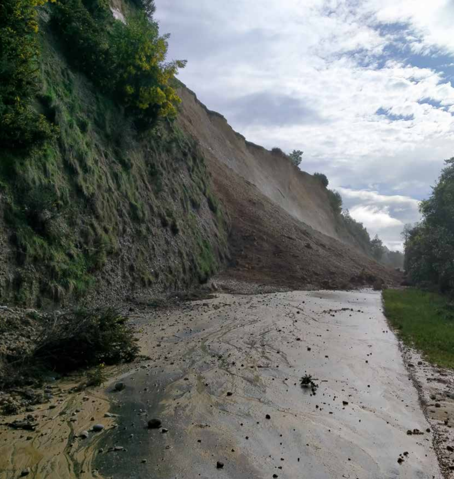
Landslide in Ruby Bay Nelson, 2022 ANNETTE LE CREN
